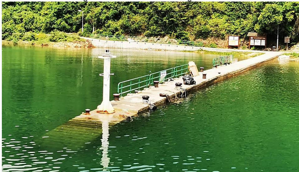
Figure 2.2: Condition of Existing LCW Pier
